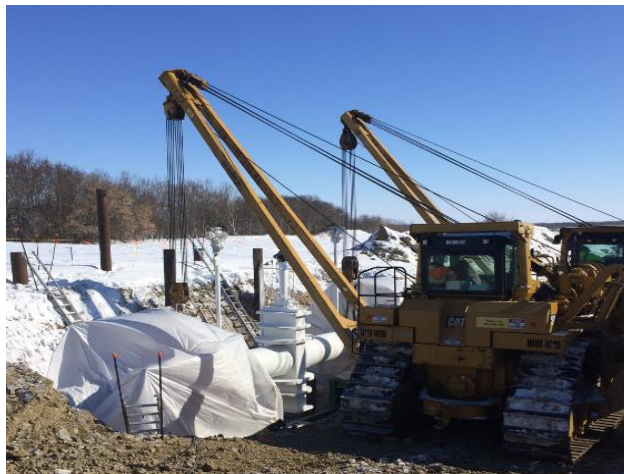
785 + 233 MLBV #22 site prepped for installation and sidebooms cradling valve at install
