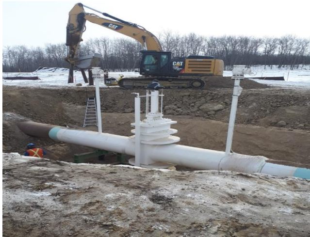
744 + 650 Crew sand shading block valve MLBV #19
