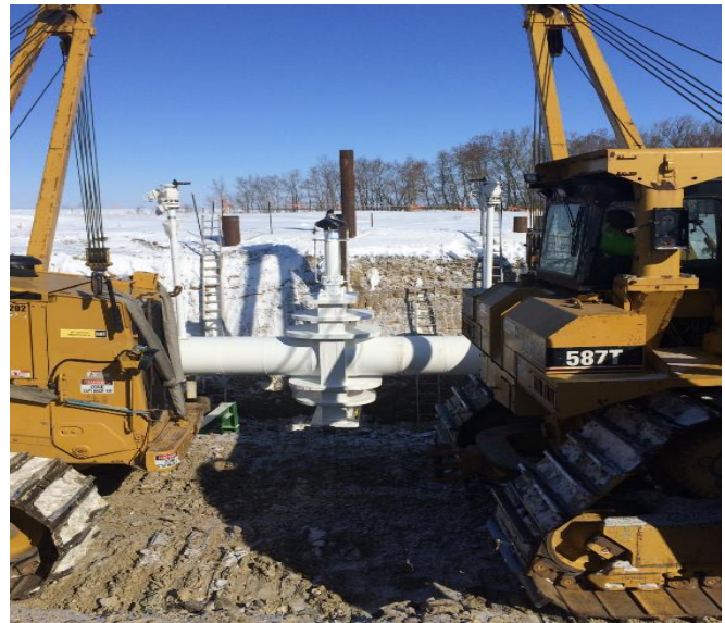
785 + 233 MLBV #22 site prepped for installation and sidebooms cradling valve at install
