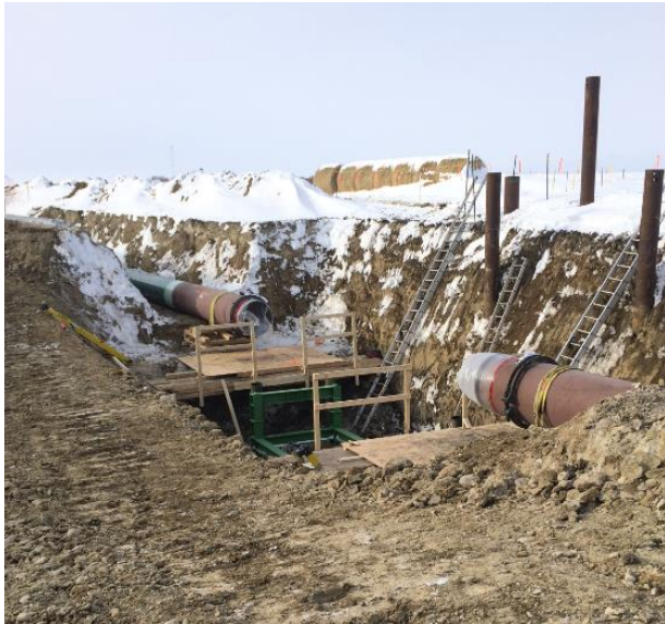
785 + 233 MLBV #22 site prepped for installation and sidebooms cradling valve at install
