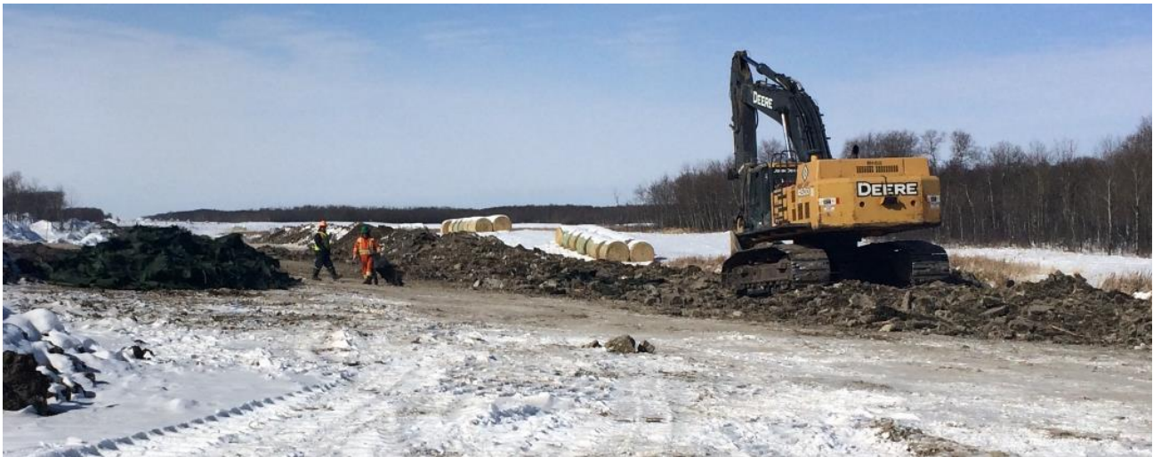
730 + 100 Ramp removal – removing geo teck SK 799
